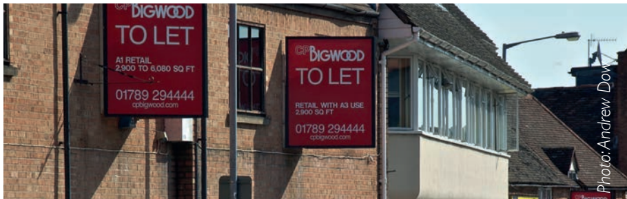
TC Project 2 Environmental Improvement Area, Greenhill Street
