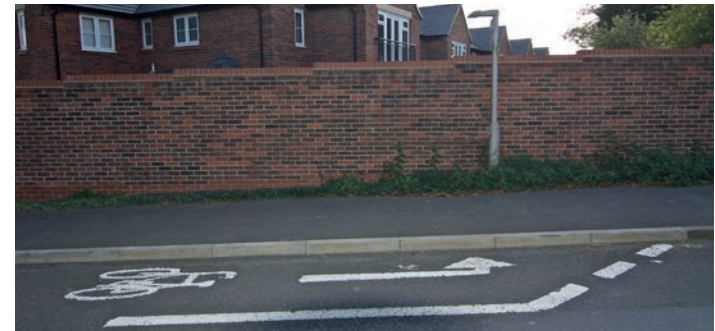
Poorly planned cycle lane, Alcester Road (above)
