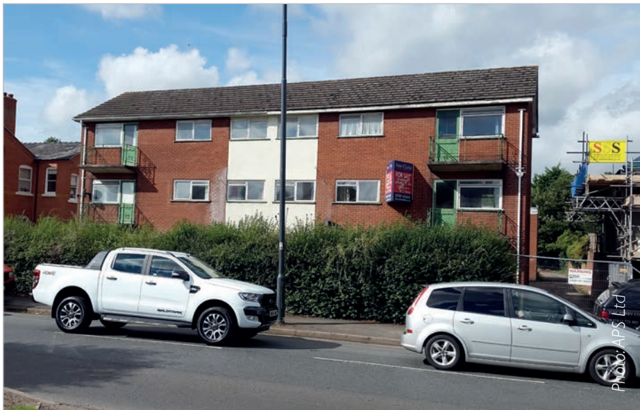
Empty Houses Shipston Road
