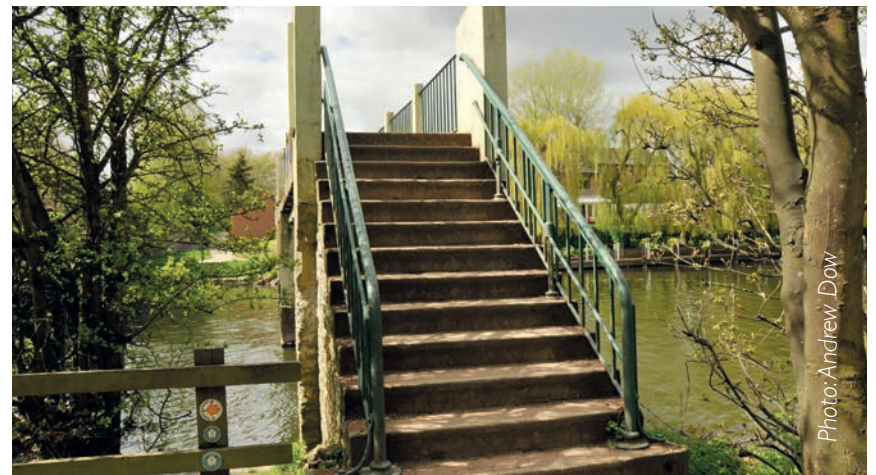
Steps at Lucy's Mill Bridge
