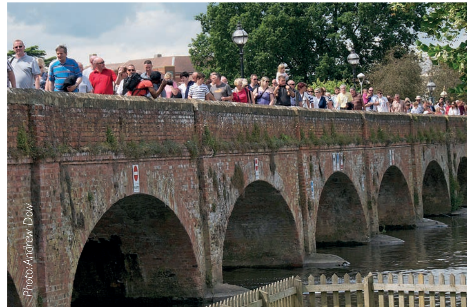
Pedestrian Congestion, Tramway Bridge
